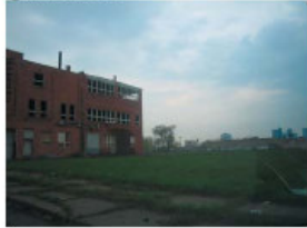
④ Vacant building
