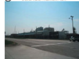
⑧ Detroit Water Treatment Plant
