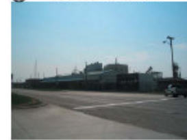
⑧ Detroit Water Treatment Plant
