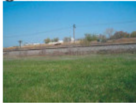
③ Downriver Wastewater Treatment Facility
